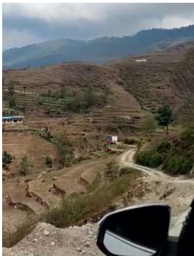
Figure 24. Access road towards substation from Baramche side
