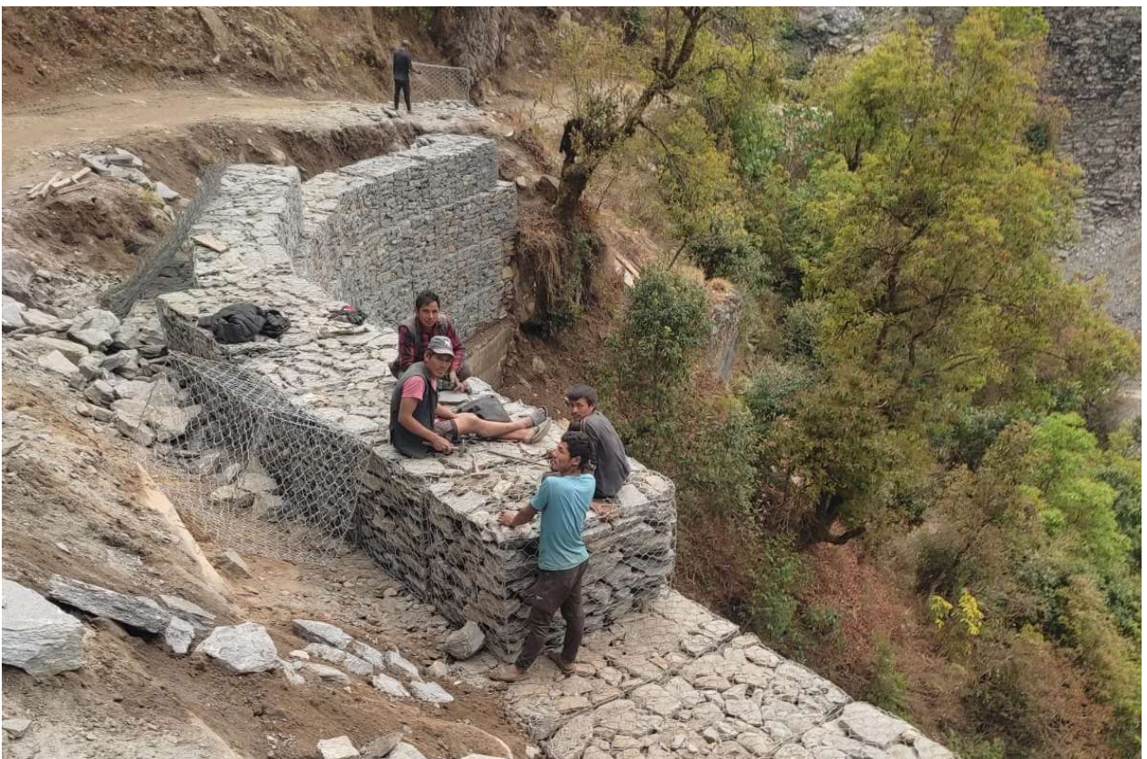
Figure 10. Upgrading access road of the project area (2023)
