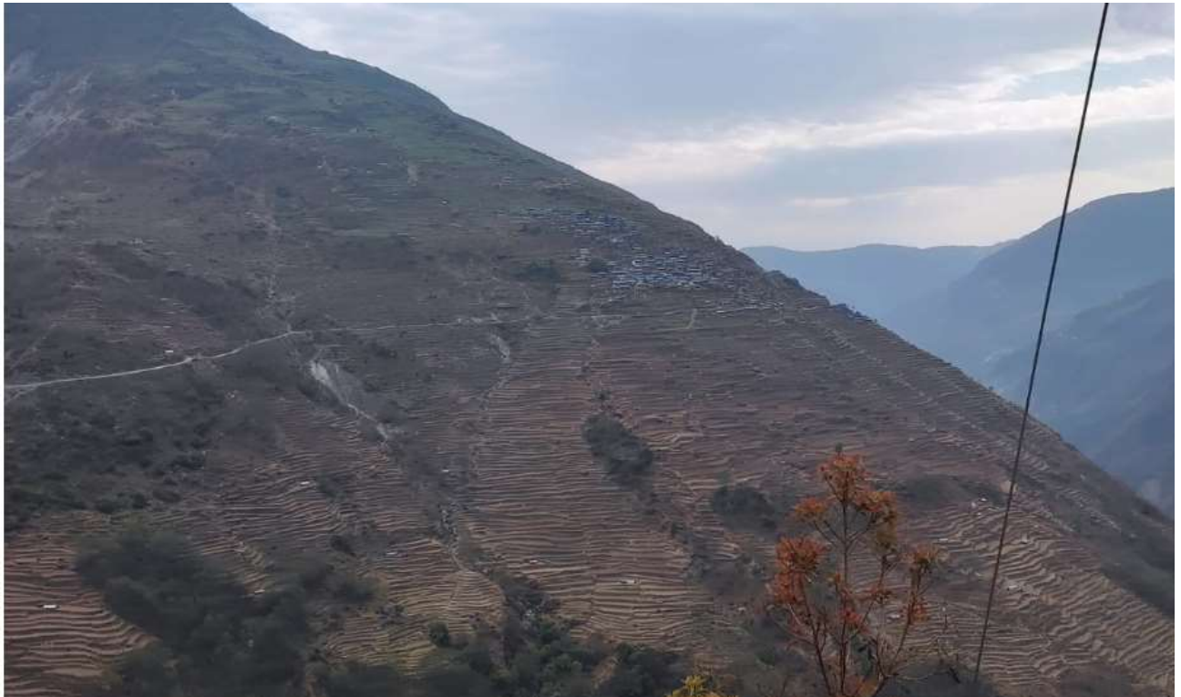
Figure 8. Access road construction of the project area by DOR (2018)
