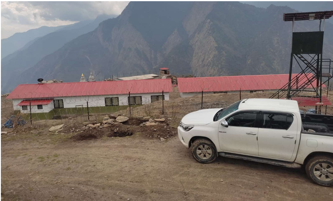
Figure 18. Army camp construction at Pokul Danda.
