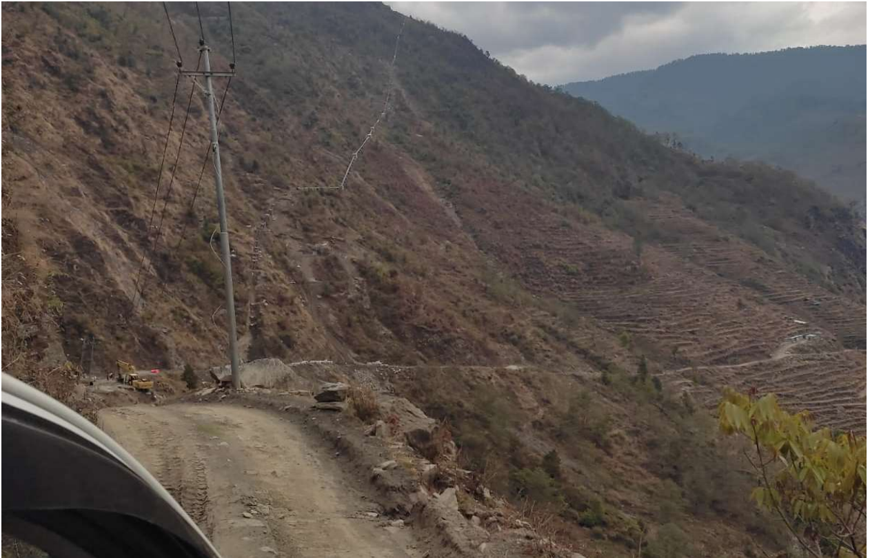
Figure 9. Access road of the project area
