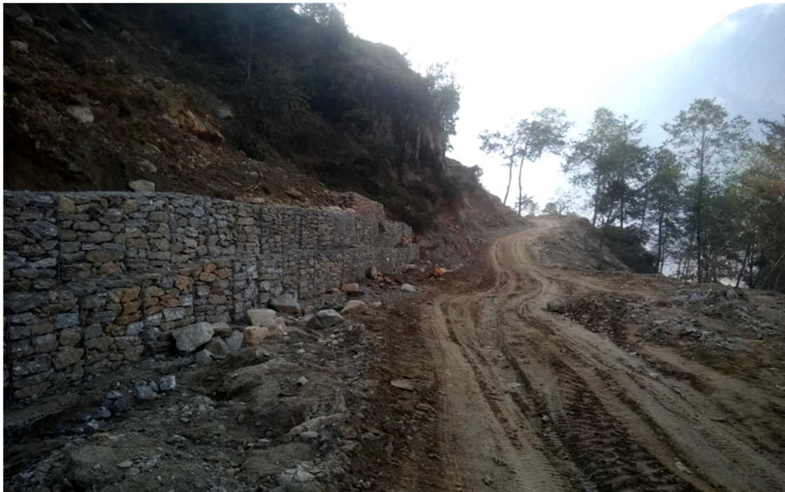
Figure 12. Access road upgrading of the project area
