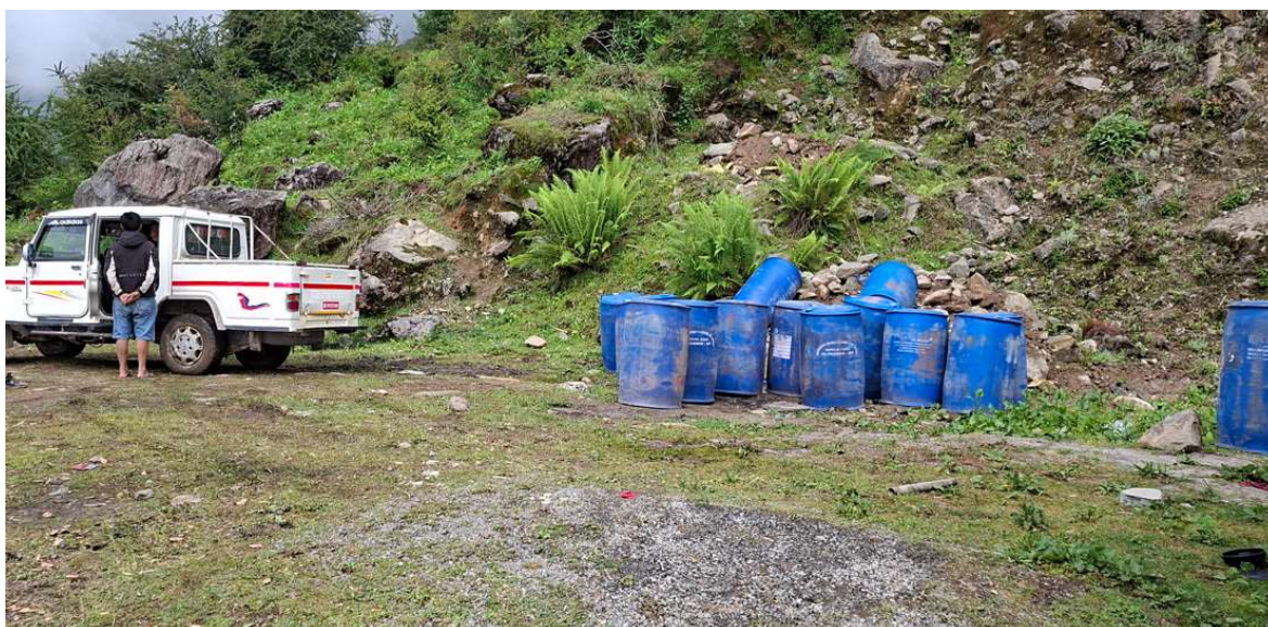
Figure 20 Fuel supply for PH excavation this month
