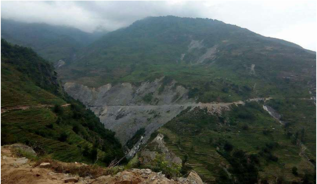
Figure 7. Access road construction of the project area by DOR (2018)
