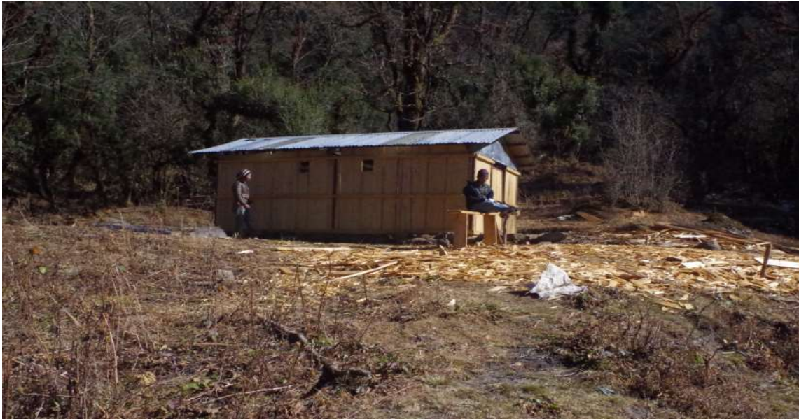
Figure 15 Camp house at Lampokhari HW
