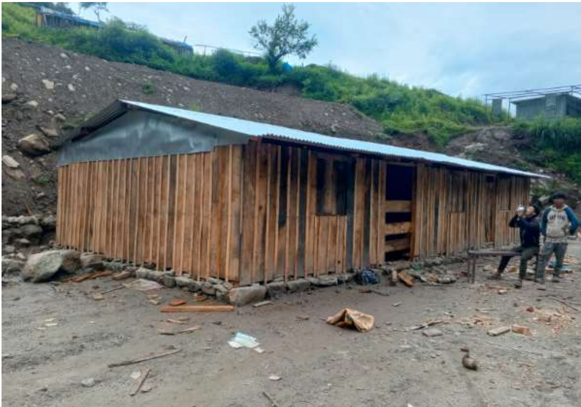
Figure 16. Camp house at -PH area at kanchasha (2025 June)
