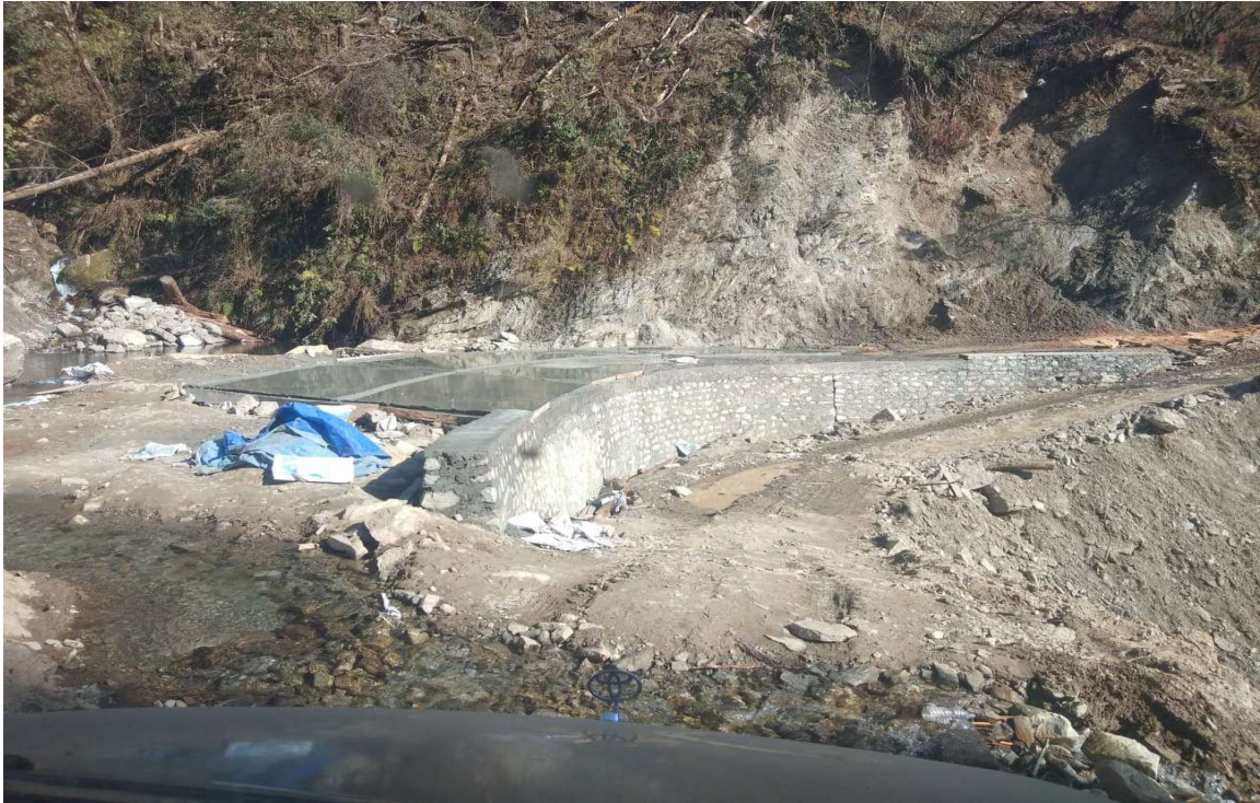
Figure 11. Access road upgrading of the project area
