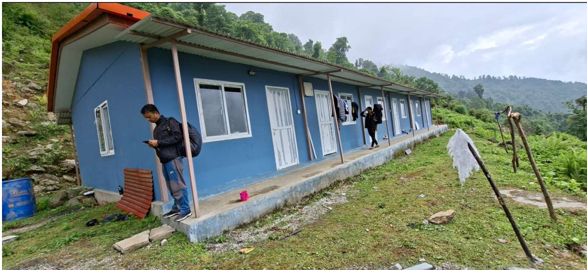
Figure 14. Camp house at Ambakharka
